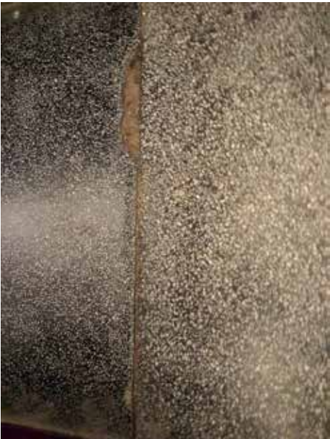
Fig. 7. Deteriorating joints and weathering of terrazzo surface in Teen Murti Bhawan, Delhi (photo by Dandona and Shah)
