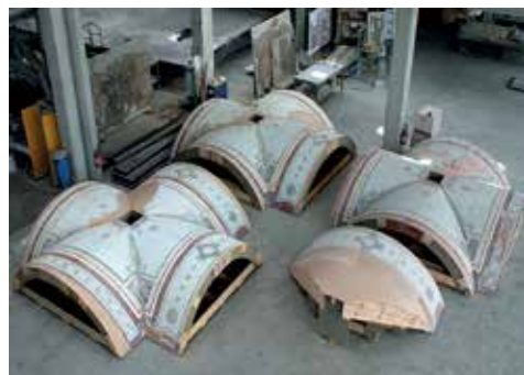
Fig. 5. Storage of vault mosaics on curved wooden supports (photo ARM)
