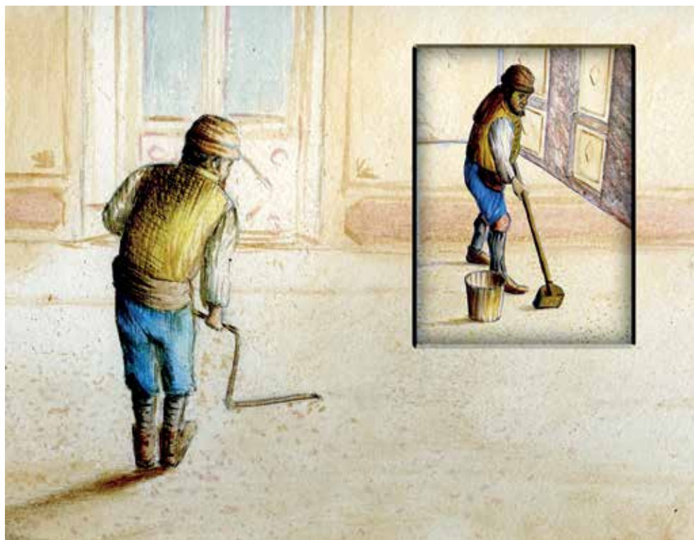
Fig. 1. Systems of beating the mortar layer and final smoothing (illustration S. Virdia)
