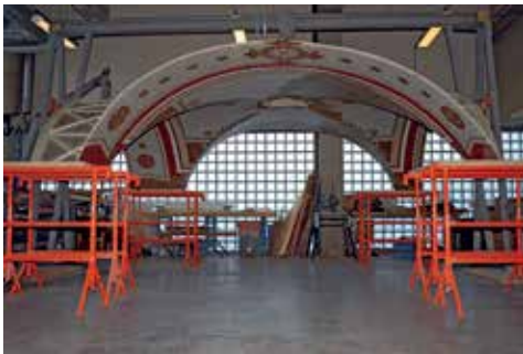
Fig. 7. Beginning of assembly of a vault in the atelier (photo ARM)
