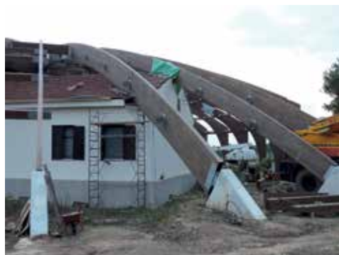
Fig. 3. Dismantling the roof of the 1930s banquet room A shelter due to errors in positioning the arch-shaped frame of new shelter (photo N. Gavrilovic, 2015)
