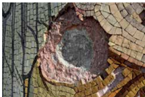
Fig. 3. Preparatory mortar stratigraphy of the Guardian angel mosaic, revealed following removal of a glass tile inserted in a shot hole, during a previous treatment. Budapest, V. József Attila u. 24 (photo B. M. Kürtösi).
