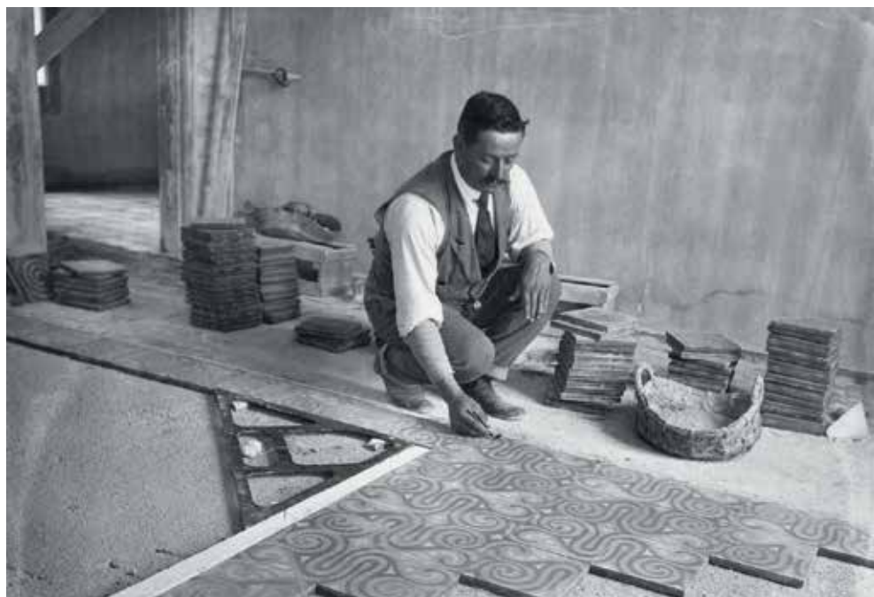
Fig. 4. Work on laying a hydraulic floor covering, image ca. 1900-1910 (Teresa Navas Collection)
