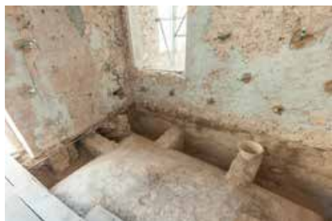
Fig. 3. Dismantling and removing the floors (photo R. Cassio)
