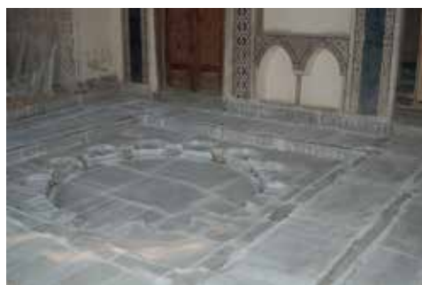
Fig. 4. Mosaics with facing, prior to extraction (photo A. Gamarra)
