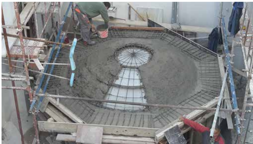
Fig. 6. Ziller-Loverdos mansion, reconstruction of the substrates (photo Hellenic Ministry of Culture and Sports)
