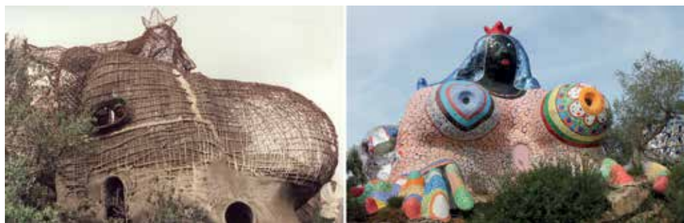
Fig. 2. The Empress-Sphinx under construction. Once the skeleton was built, it was covered by a layer of concrete using spritz beton technique, and by an additional layer of lighter concrete. The form was then decorated with ceramic, glass and mirror tiles (photo S. Vella)
