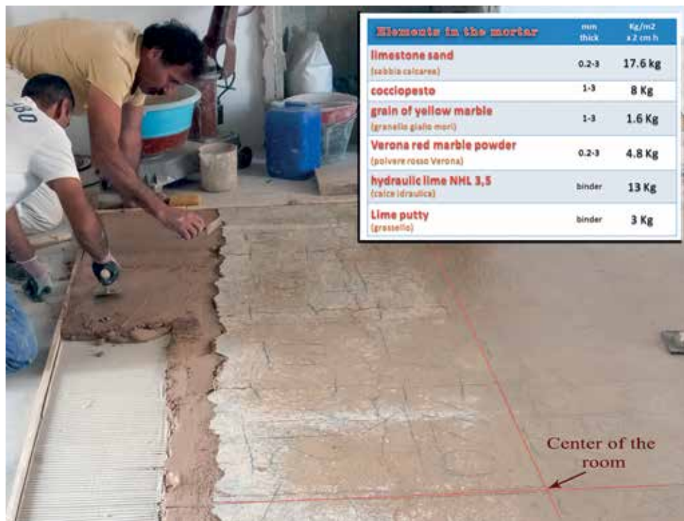
Fig. 9. Re-laying the terrazzo on site (photo R. Cassio)
