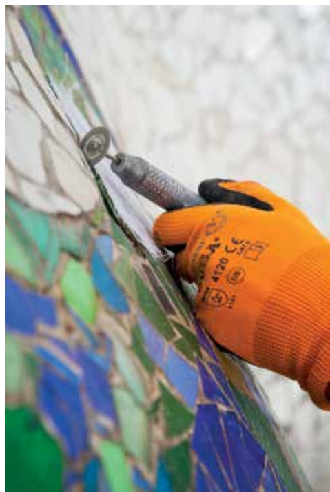
Fig. 5. Cutting using micro-tool with diamond blade (photo M. Fábregas, La Fotografica)
