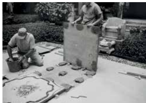
Fig. 8. Levelling mosaic panels on cement pads, 1961 (ISGM, photo J. B. Pratt)
