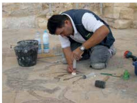
Fig. 8. Consolidation by injection of the mosaic of the Diaconicon Baptistry (photo Franco Sciorilli)
