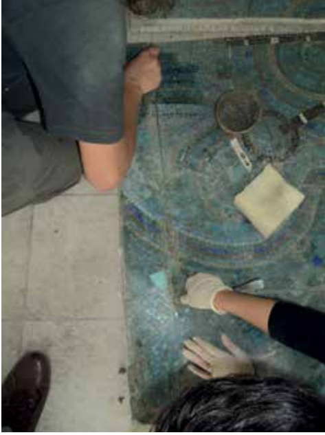
Fig. 8. Application of joint filler to the tessellatum (photo S. Şener)
