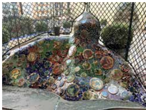
Fig. 4. Final cleaning posterior to regrouting the glass trencadís and ceramics elements (photo N. Zapata)
