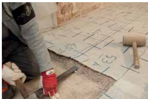
Fig. 5. Using chisels to detach the uppermost layer of mortar (photo R. Cassio)
