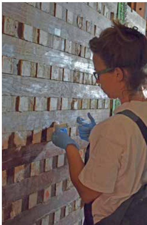
Fig. 10. Injecting grout for consolidation of the support (photo Atelier de conservation-restauration, Musée départemental Arles antique)
