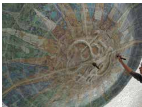
Fig. 3. Application of facing and marking of cut lines between sections (photo Gamarra & Garcia)
