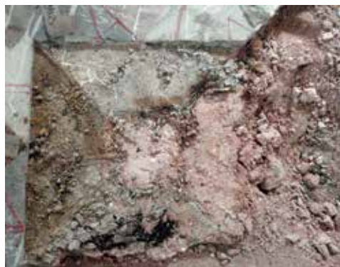
Fig. 1. Example of use of many different mortars for the floor of the sanctuary (photo E. Pannunzio)
