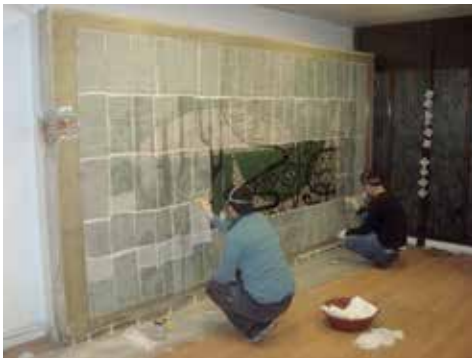
Fig. 3. Application of temporary facing (photo S. Şener)
