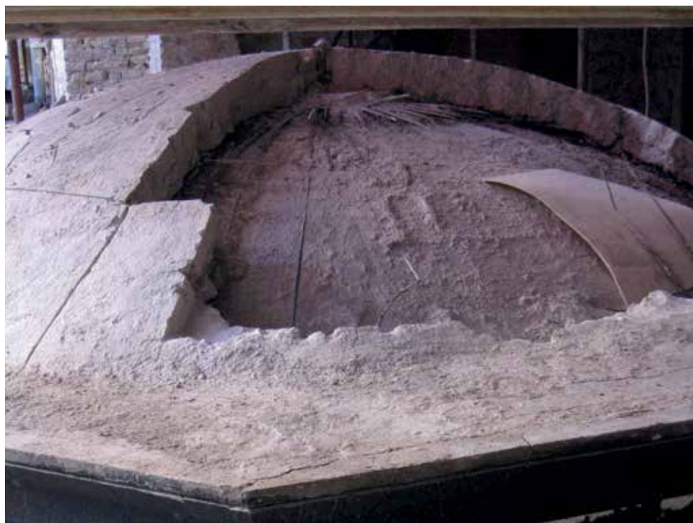
Fig. 5. Ziller-Loverdos mansion, vault mosaic, severe damage of mosaic substrates (photo Hellenic Ministry of Culture and Sports)
