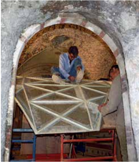
Fig. 9. Reinstallation of re-backed modules in the crypt (photo ARM)
