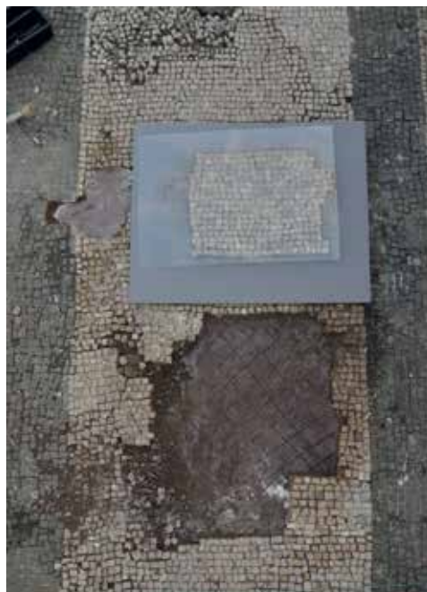
Fig. 3. Intervention of restoration: mosaic detachment and replacement operations, indirect method (photo by A. Borzomati)
