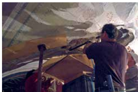
Fig. 4. Removal of vault mosaics (photo ARM)
