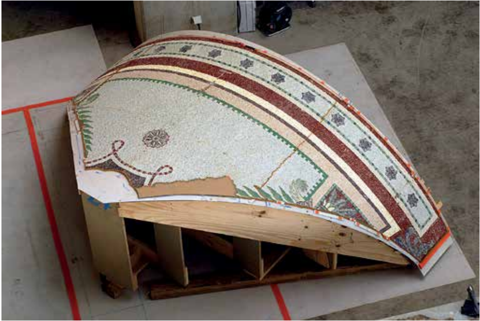
Fig. 6. Reverse side of tessellatum after assembly of modules composing a vault quarter (photo ARM)
