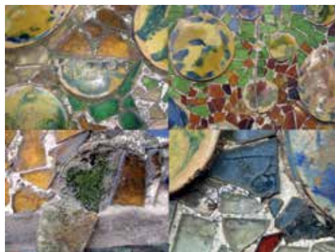
Fig. 2. Deep cracks, biological growth and loss of glass trencadís (photo N. Zapata)
