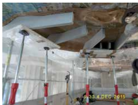
Fig. 4. Making a mould using thermoform sheeting and polystyrene (photo Gamarra & Garcia)
