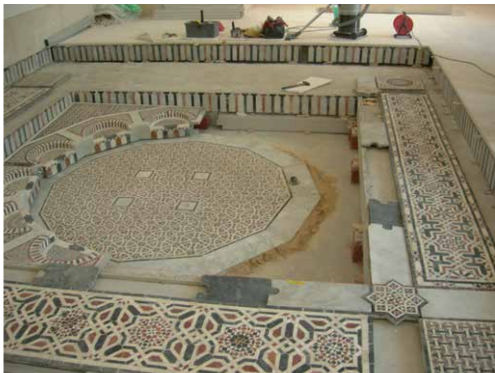
Fig. 8. Installation of the pieces of the fountain in their new location at the MIA (photo A. Gamarra)
