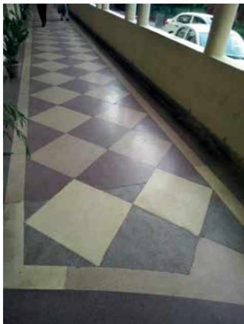
Fig. 5. Patching of terrazzo in All India Radio (Broadcasting House), Delhi (photo by Dandona and Shah)
