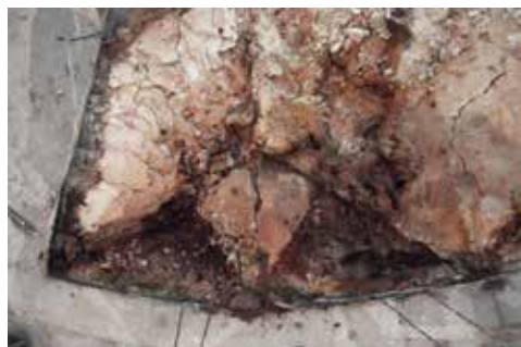
Fig. 2. Mortar using resin and white lime binder for the laying of the altar tarsia (photo E. Pannunzio)
