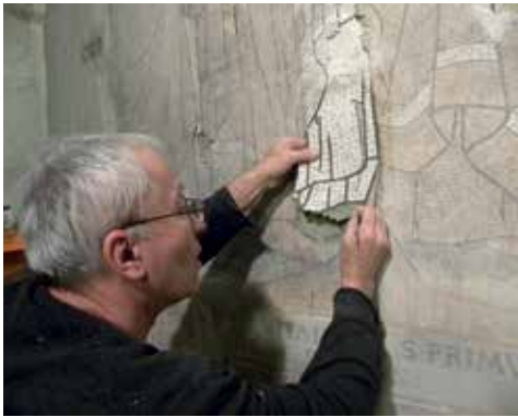
Fig. 10. Re-fitting a lifted fragment on lime mortar (photo ARM)
