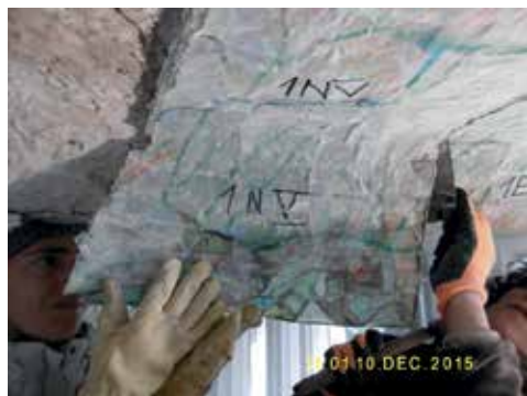
Fig. 6. Detachment of a mosaic section (photo Gamarra & Garcia)
