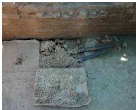
Fig. 10. Detachment of an area of irregular terrazzo (photo K. Schneider and F. Guiducci)
