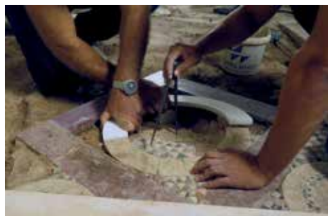
Fig. 6. South panel, during positioning of new marble elements (photo I. Doganis)
