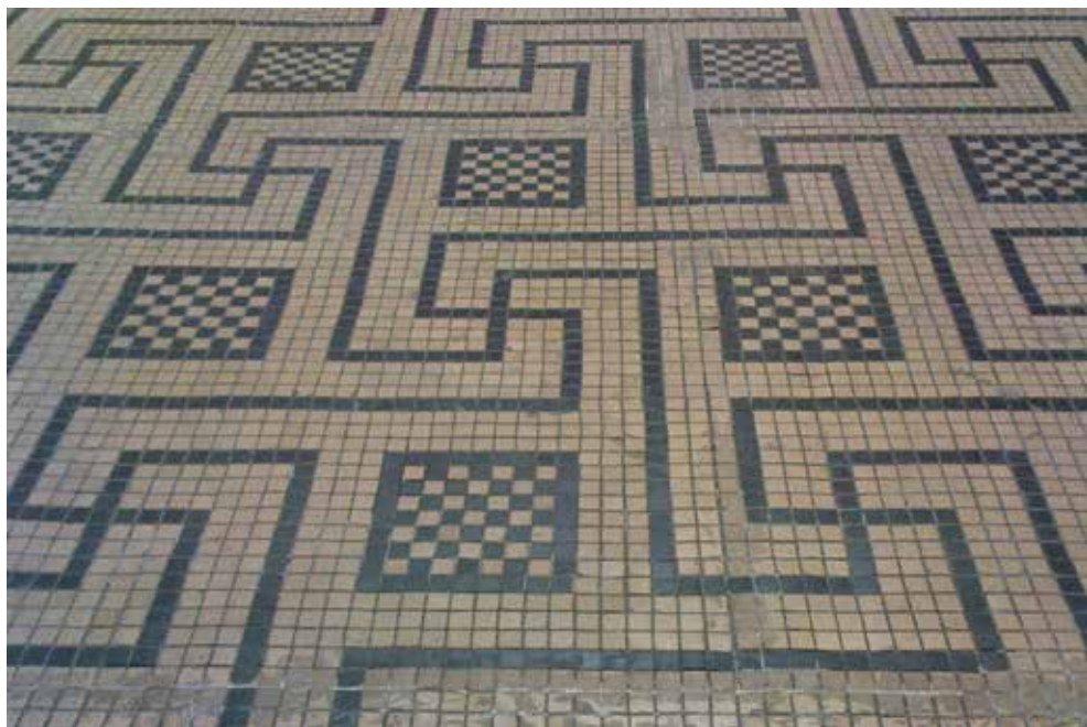
Fig. 9. Detail of precast ceramic tesserae mosaic in the lobby of Pallas theatre, ex- Army Share Fund Building, constructed 1928-1940 (photo by L. Tapini)
