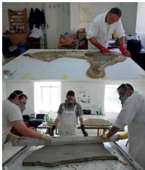
Fig. 4. Preparation of the mosaic support: a) application of NHL mortar; b) application of epoxy resin mortar
