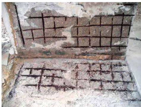
Fig. 1. The oxidation of the metal reinforcement bars in a concrete mosaic backing (photo A. Ouslati)
