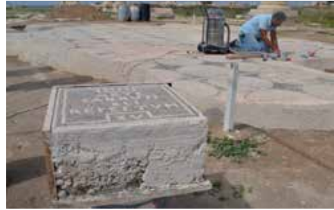
Fig. 3. Demonstration piece showing the substrate reconstruction, with inscription ARTE FABRVM XLI REFECTVM, signifying the restoration by the skill of forty-one artisans (photo Badde/MacKinnon 2014-2016)
