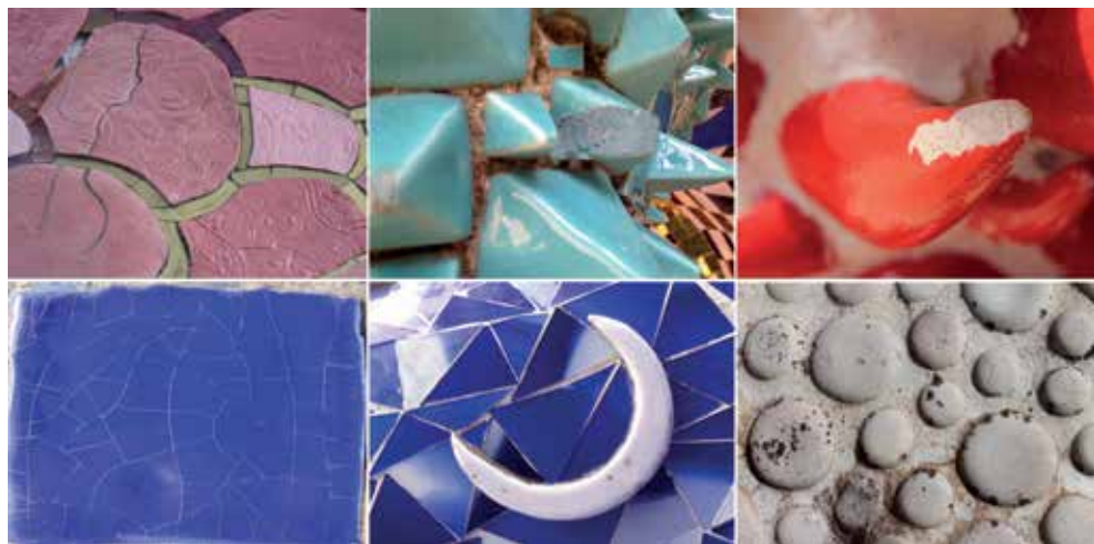
Fig. 4. Left to right: cracking of the surface materials; cracking and loss of the ceramic glaze; cross linking of the ceramic glaze; abrasion of the gold glaze, biological attack (photo S. Vella)
