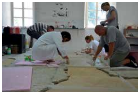
Fig. 8. Application of the decorative mortar to mosaic panels
