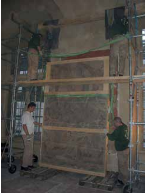
Fig. 4. Removal of the Neptune and Amphitrite mosaic from the wall of the Mosaics Gallery in 2007 (photo Musée du Louvre/Cécile Giroire)
