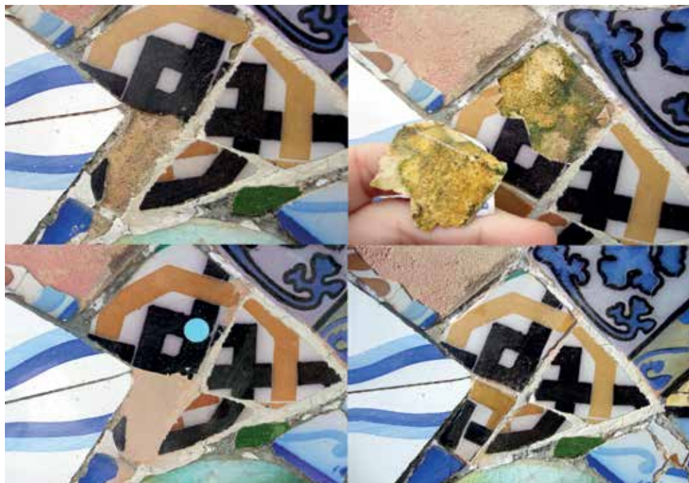
Fig. 3. Separation of glazing, cleaning, consolidation and final results, 2016 (photo A. Cusó)
