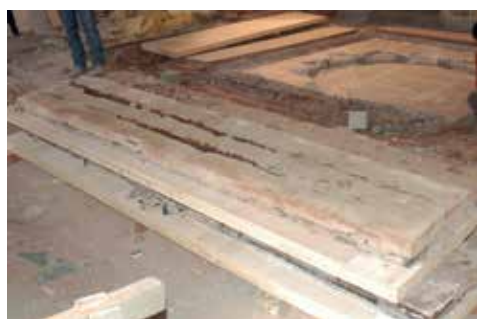
Fig. 5. Removal of the blocks supporting the mosaic, showing effects from iron oxidation (photo E. Porta)
