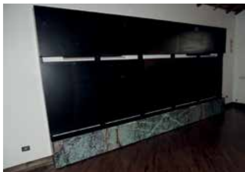
Fig. 9. Arcinazzo Romano, Villa of Emperor Trajan: antichamber , construction of the steel wall for the west wall of room XXV (photo by A. Lugari)
