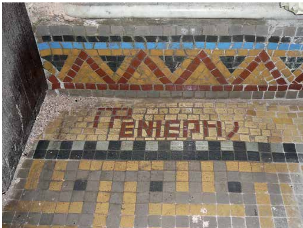
Fig. 8. Detail of signature on precast ceramic tesserae, Loverdou - Ziller mansion (photo by L. Tapini)
