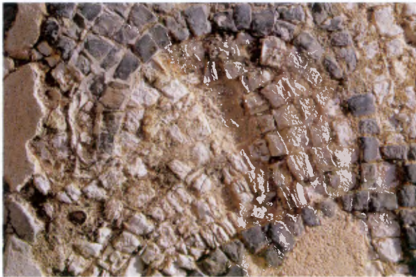
Fig. 5 : Sabratha. The theatre baths. Detail of the mosaic floor in the southern apodyterium : the crumbling of the tesserae .
