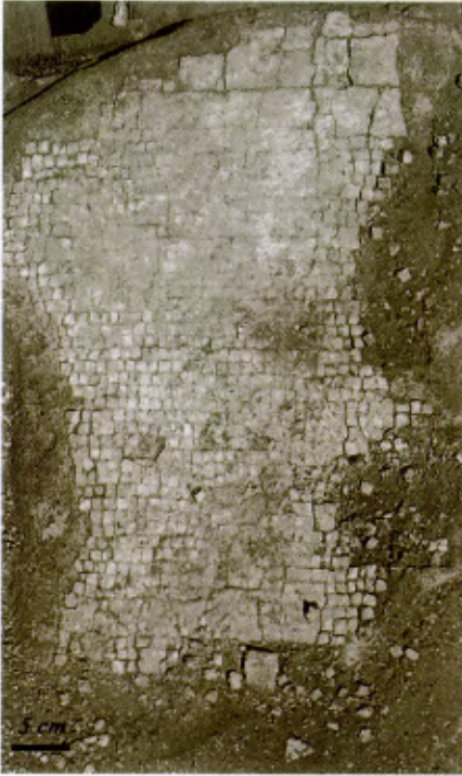
Fig. 4 : This small mosaic is not part of the test. The mosaic is located in a zone where visitor to the sites passes by. The mosaic is in unstable condition with loose tesserae and damaged borders.
