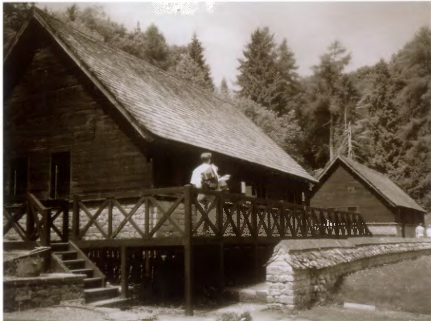
Fig. 1 : View of two of the mid 19th enclosures over the mosaics.
