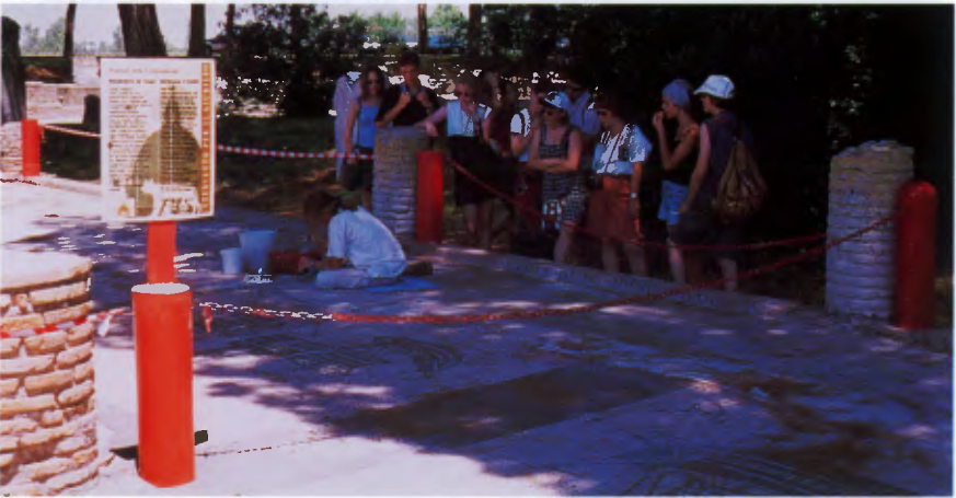
Fig. 2-3 : Ostia Antica, Piazzale delle Corporazioni. The materials used for cleaning the mosaics were water, mechanical and manual strength. Slaked lime, sand and stone powder were used for relaying tesserae. Hydraulic lime Lafarge and stone powder were used for consolidation between the tesserae.
