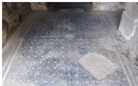
Fig. 16. Mosaic floor of the peristyle corridor 18 with extensive abrasion and mortar repairs, Casa del Salone Nero, Herculaneum (May 2011) (photo: Niki Savvides)
