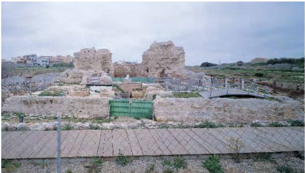
Fig. 1. The monumental complex of Palazzo Re Barbaro in the first phase of intervention on the peristyle. View from the north (© Soprintendenza Archeologica per le province di Sassari e Nuoro)
