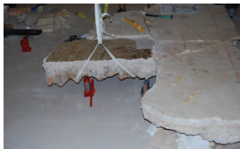
Fig. 6. Positioning of the different parts using small, high precision lifting mechanisms (photo: Chr. Pilalis)
