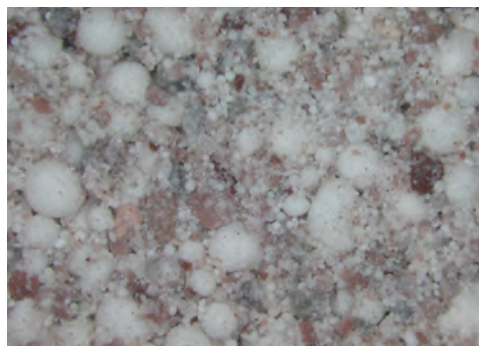
Fig. 8. The new lime-based mortar with light-weight aggregates (glass foam products) (Photo: Brigitta Maria Kürtösi)
