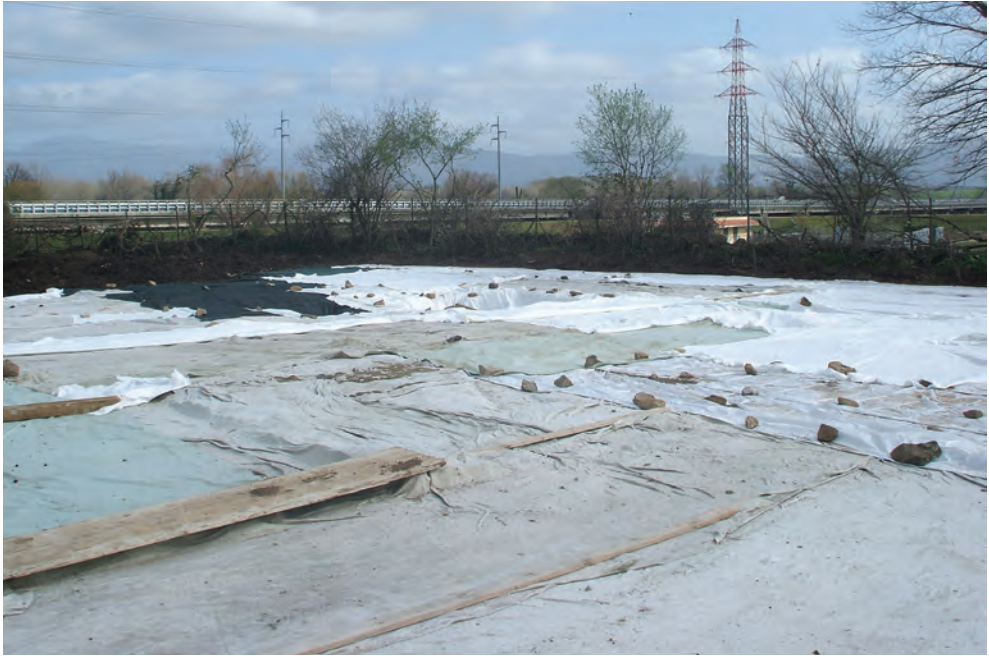
Fig. 1. Covering mosaic floors with nonwoven fabric, Villa Fontana Amara, Rome (photo: A. Lugari)
