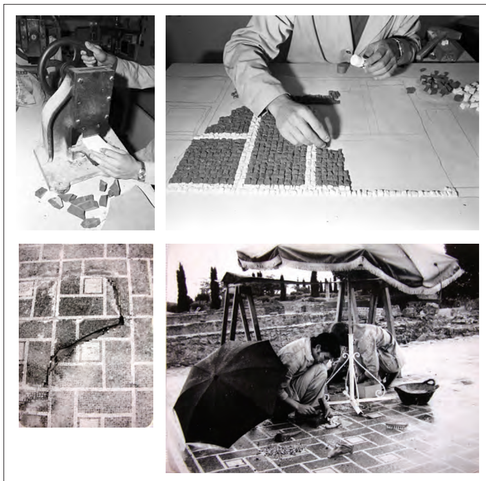
Fig. 7. Lacunae reintegration (in the 1970s) in area 9 of Domus 2A in the Roman City (photos: Mac-Empúries Archives)
