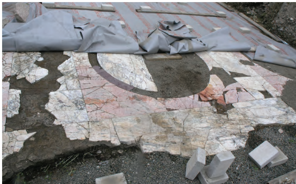
Fig. 6. Condition after one year of covering with Delta-Lite fabric, Forum of Peace, Imperial Fora, Rome (photo: A. Lugari)
