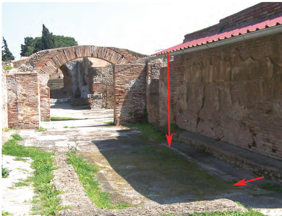
Fig. 2. Increase of the biological cover linked to a higher input of water and earth arising from a nearby shelter (photo: G. Caneva)
