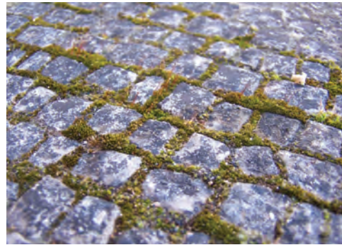
Fig. 4. High moss colonization in the interstices between the tesserae (photo: S. Brignocchi)
