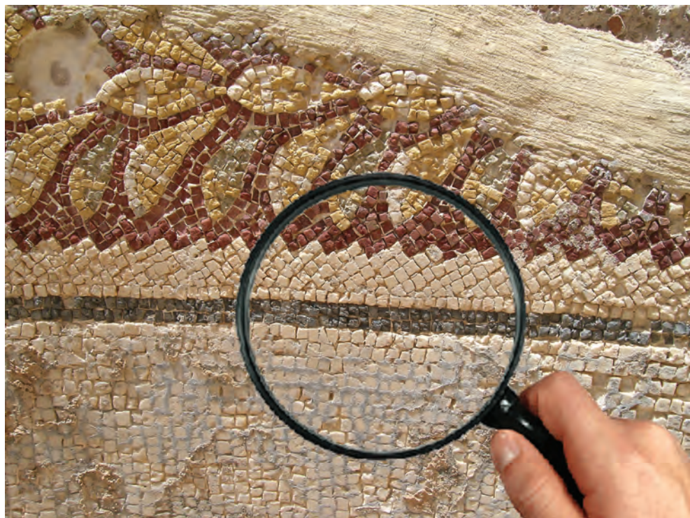
Fig. 1. The level or depth of inspection of a mosaic condition survey depends on specific circumstances and objectives. The amount of survey information previously gathered, the significance of the mosaic, its condition and risk environment all inform the level of survey that is appropriate for a particular case (© John Stewart)
