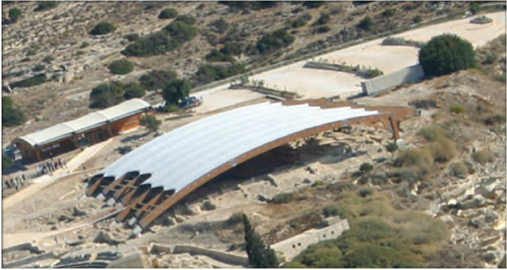
Fig. 4. Kourion, the shelter over the “House of Eustolios” (photo: E. Charalambous/ Department of Antiquities of Cyprus)
