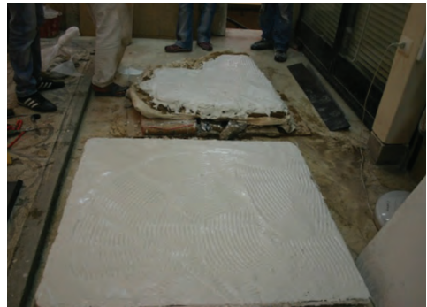
Fig. 10. Putting the mortar on the board and panel
