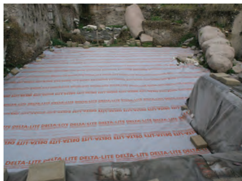
Fig. 8. Covering with a 'single' sheet of Delta-Lite fabric, Forum of Peace, Imperial Fora, Rome (photo: A. Lugari)
