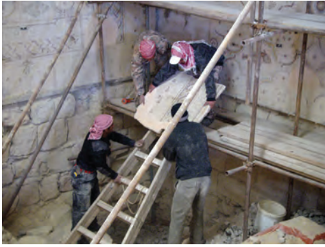
Fig. 7. The removal of the mosaics for their restoration, February 2008 (© C. Pappalardo)
