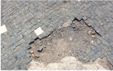
Fig. 18. Lacuna on peristyle corridor 16, Casa del Salone Nero, located close to the tablinum with a deteriorated battuto , from where gravel is transferred onto the mosaic and may be related to the losses affecting the floor (May 2011) (photo: Niki Savvides)
