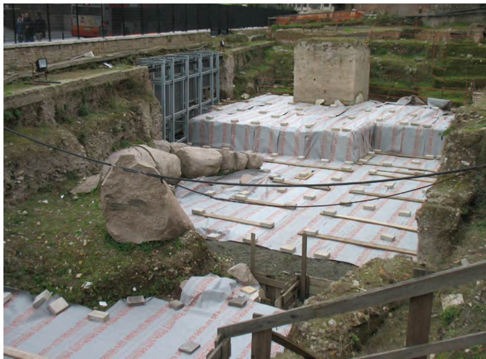
Fig. 5. Covering with Delta-Lite fabric, Forum of Peace, Imperial Fora, Rome (photo: A. Lugari)
