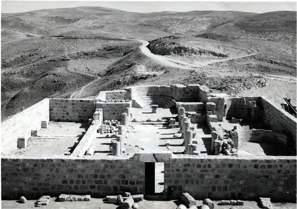
Fig. 3. The perimeter walls of the Memorial repaired to be reused for the shelter, 1964 (© SBF, Jerusalem)
