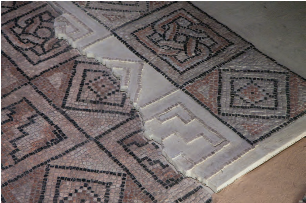
Fig. 6. This reintegration technique in the Domus dei Tappeti di Pietra, Ravenna, Italy, is at a higher level than the mosaic surface. Looking at the mosaic from above it seems as if they are at the same level (photo M. Kindt M., 2012)
