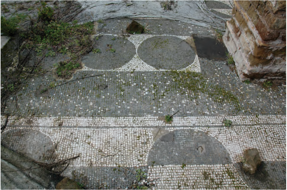
Fig. 3. Condition after one year of covering with nonwoven fabric, Villa di Via Carciano, Rome (photo: A. Lugari)
