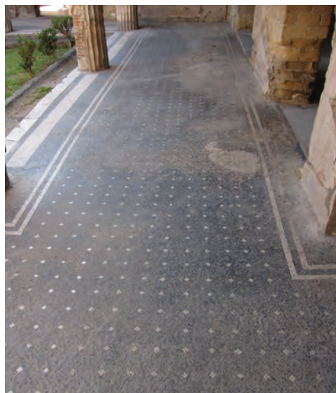
Fig. 16. Mosaic floor of the peristyle corridor 18 with extensive abrasion and mortar repairs, Casa del Salone Nero, Herculaneum (May 2011) (photo: Niki Savvides)
