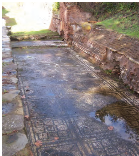
Fig. 3. High growth of algae and cyanobacteria in humid conditions (photo: S. Brignocchi)
