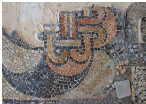
Fig. 15. The material of the new tesserae supplements was a geologically similar massive limestone. The lime-based VAPO inject 01 was used as bedding mortar (Photo: Brigitta Maria Kürtösi)
