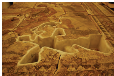
Fig. 7. Edging the lacunae of the mosaic into the gaps (photo: Chr. Pilalis)
