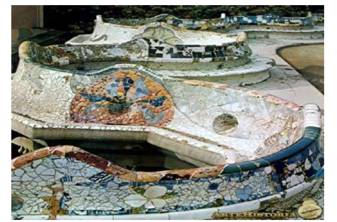
Deterioration state before replacement of pieces
