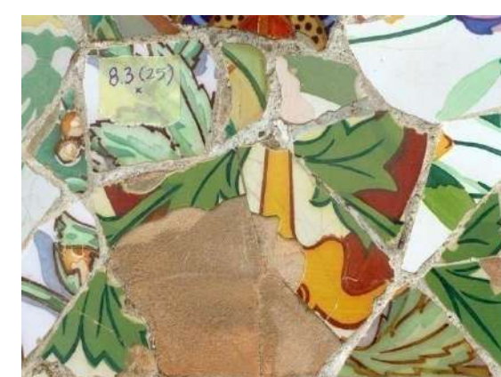
Section 35-36, deteriorated trencadís
