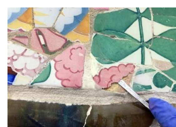
Section 44, separation of glazing elements
