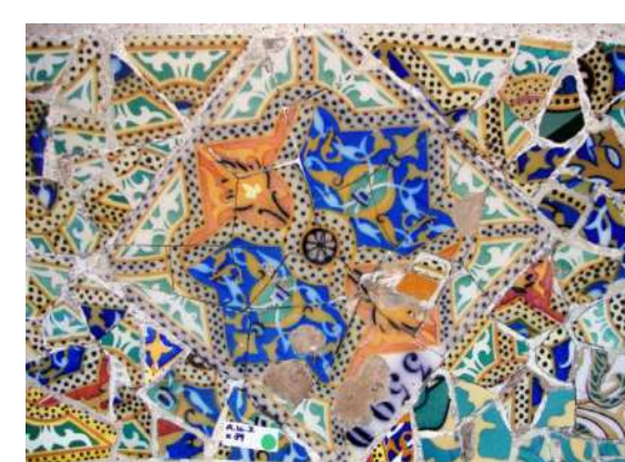
Section 35-36, deteriorated trencadís
