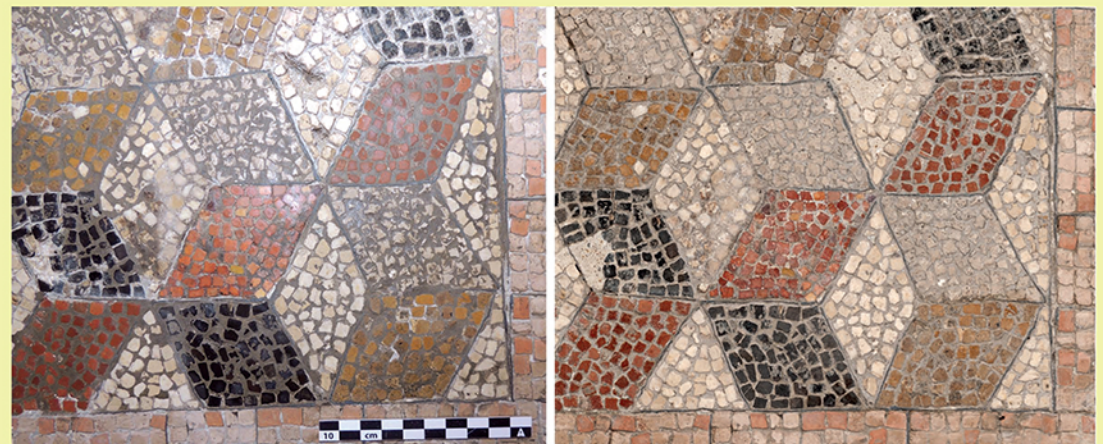
Detail of pavement before and after removal of the cement
