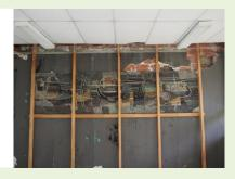
Two contemporary mosaics made in 1967 by the french artist Camille Hilaire have to be protected, transferred and restored in new rooms of an highschool in Creutwald (Eastern France). As they are made on asbestos supports, the removal has to be very careful. A team with asbestos specialists, metalworking craftsman and conservator has been created.
