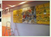
Once on place, surface protections are removed and the last operation of cleaning and reintegration of tesserae is done. A new join is applied to cover the cracks and the junctions between panels. All the periphery of mosaics is covered by a mortar to isolate asbestos on each side. A new lightening system "bring the mosaics to light" in the highschool.
