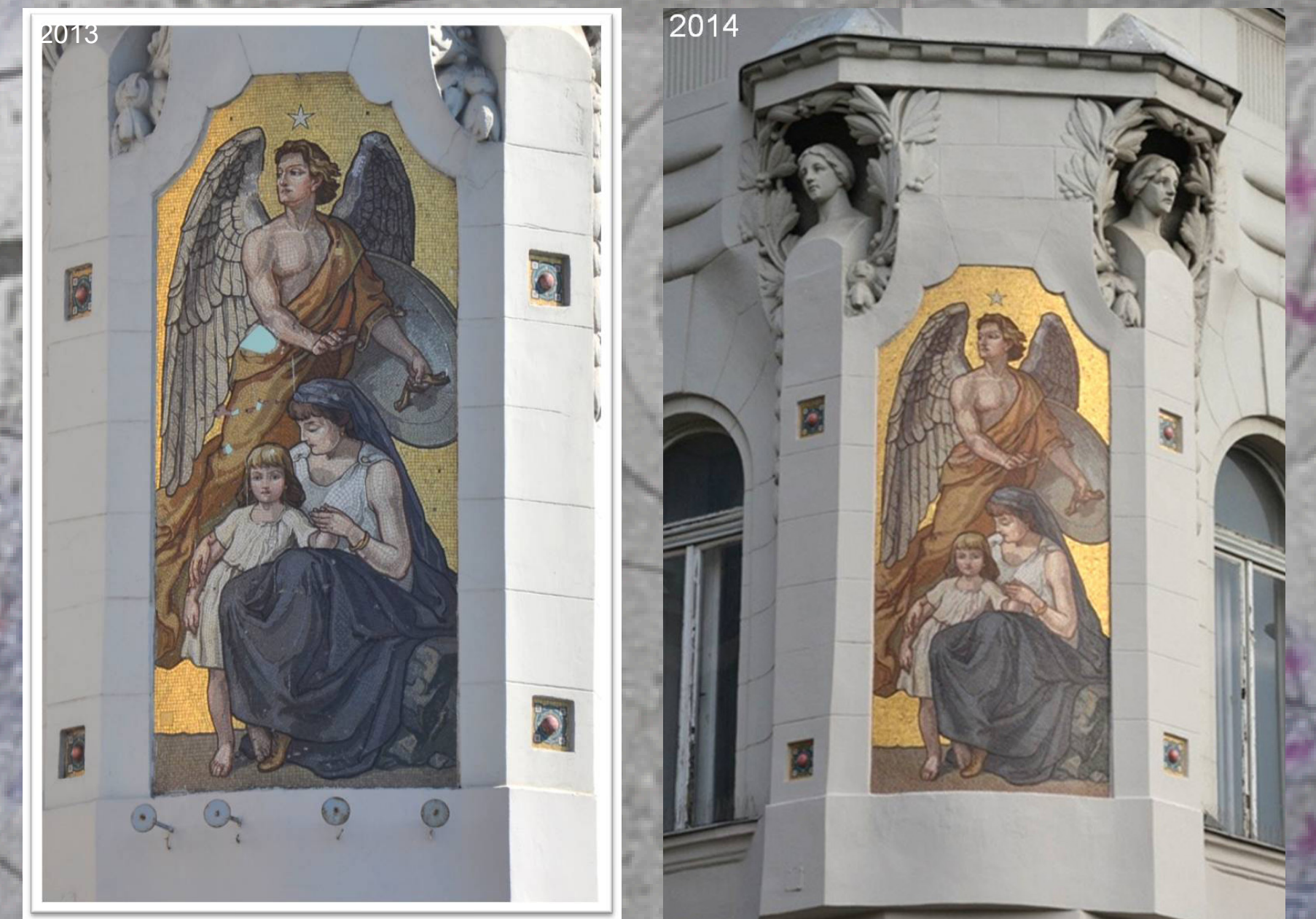
The common technique is a several cm thick brick wall built for wearing a couple of mortar layers. The mortars were lime-based ones, with sharply crushed limestone in different fractions added. The colour of these mortars has a pinkish hue.
