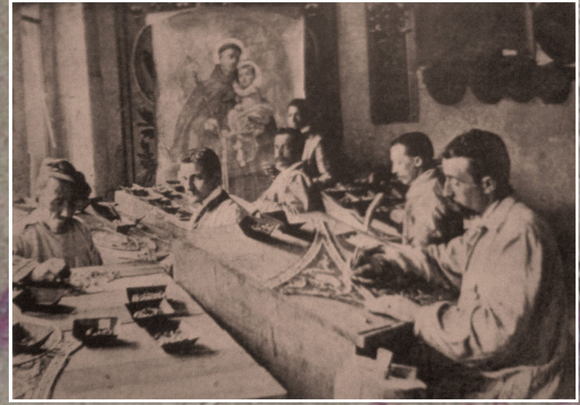
The mosaic was creating in the studio and its units were mounted on the spot by the help of temporary support. In many cases the meeting boundaries of the units can be observed.
