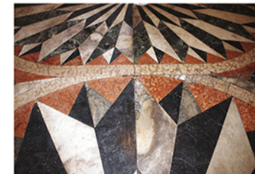
Altar front side: where the floor is isolated from the building structures, the stone slabs are in quite good conditions. Fractures and deformation occurred just alongside the steleri edges.
