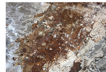
Altar left side: rosin mixture state of preservation. The vegetal resin was the only original binder found while gypsum and concrete mortars were employed during several maintenance past events.
