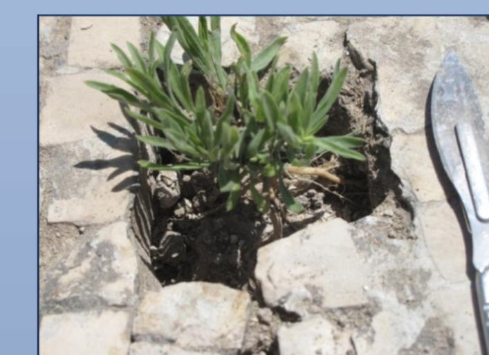
Mechanical removal of the weeds, grasses and bushes is done by removing some tesserae to be able to extract roots.
