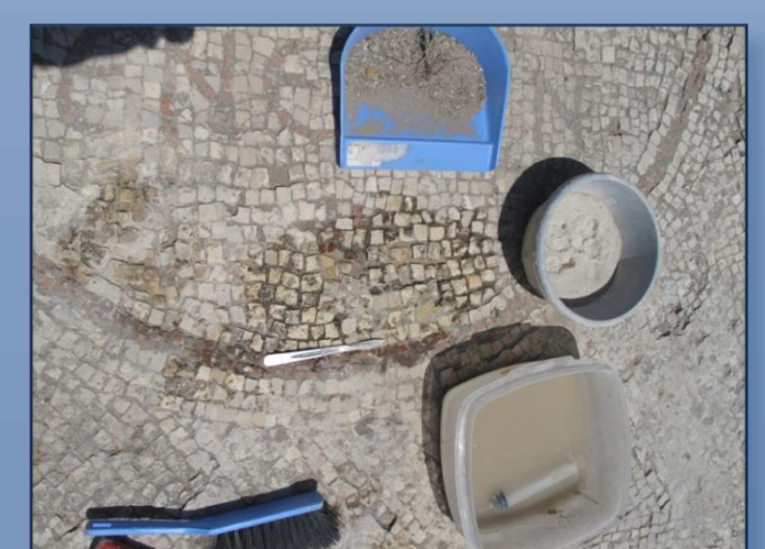
Resetting tesserae, consolidation and filling gaps are done by using hydraulic lime mortar.
