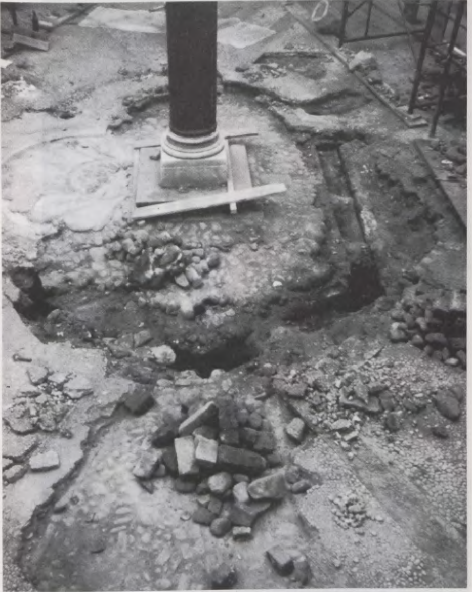
Fig. 8 - Court of the Rains : test dig to locate the pipes and their waste wells
