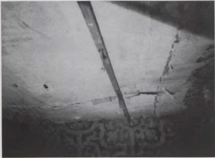
Fig. 5a - Room of deformed wall: horizontal cuts in the mosaic surface Fig. 5b - Room of deformed wall: deformed mosaic repositioned by means of wooden planks
