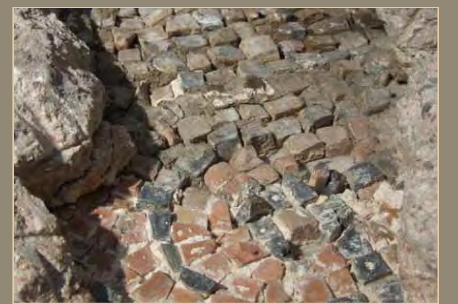
The back of the original tesserae with traces of the white bedding mortar ( below ) and the later supplement in cement ( above )
