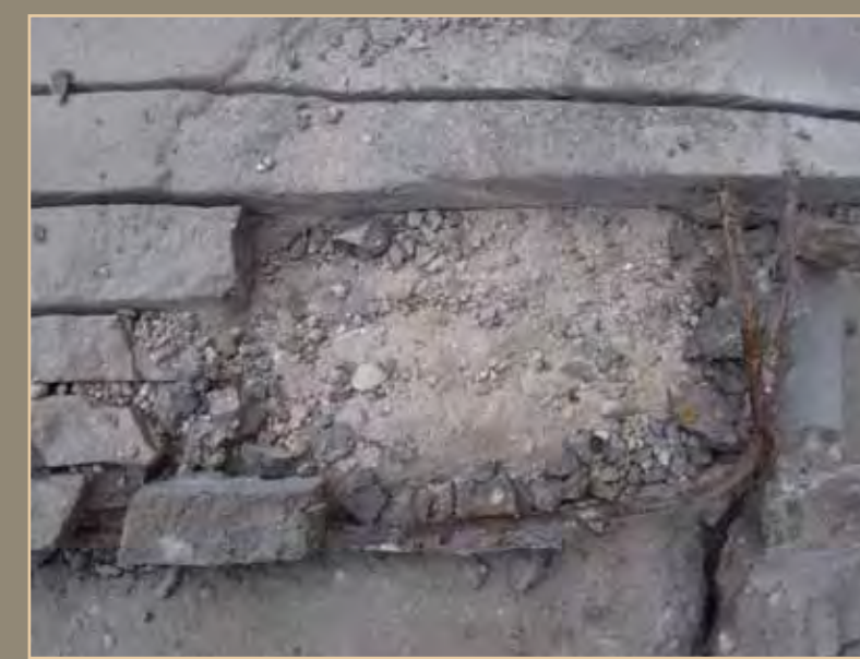
The removal of the concrete support
