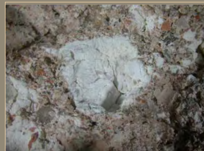
"Kalkspatzen" - detail of the first layer of the nucleus
