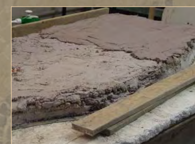
Levelling of the backside of the mosaic was made by the lightweight lime-based mortar ( above )
