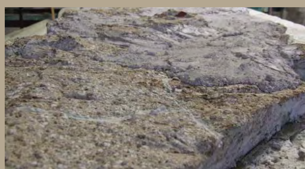
The back of the fragment with the original and the new mortar
