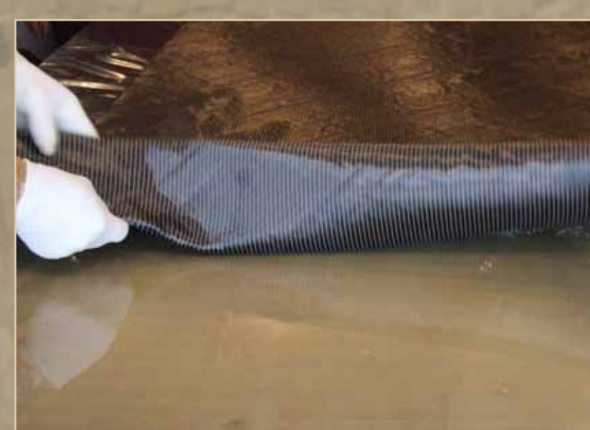
The preparation of the new support with woven carbon fibre and 3PSP2 resin
