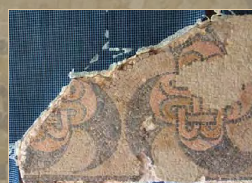
The place of the entirely missing parts was formed by 6 cm thick glass foam panels, glass net and a thin layer of lightweight lime-based mortar
