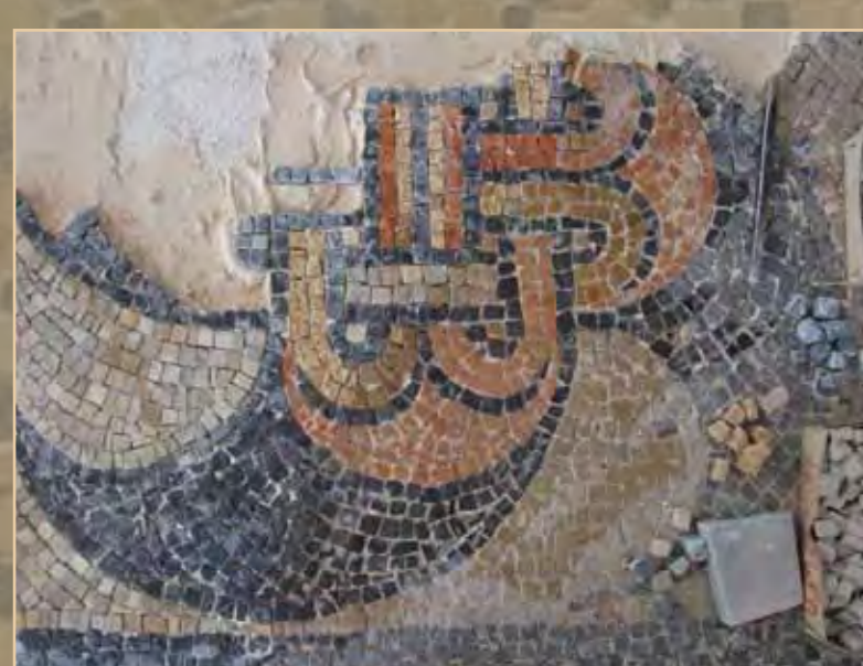
The material of the new tesserae supplements was geologically similar massive limestone. The lime-based VAPO inject 01 was used as bedding mortar
