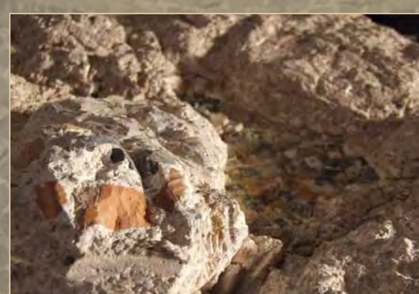
The level differences of the remained mortar layers were 6-10 cm
